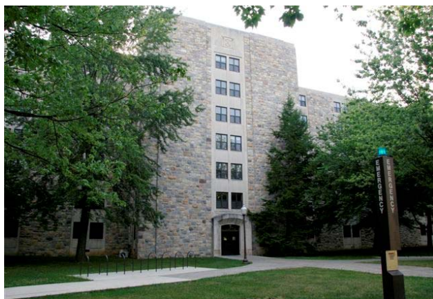
Figure 3. Exterior of West Ambler Johnston
