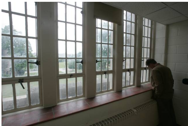
Figure 11. Typical Set of Windows in Norris Hall
