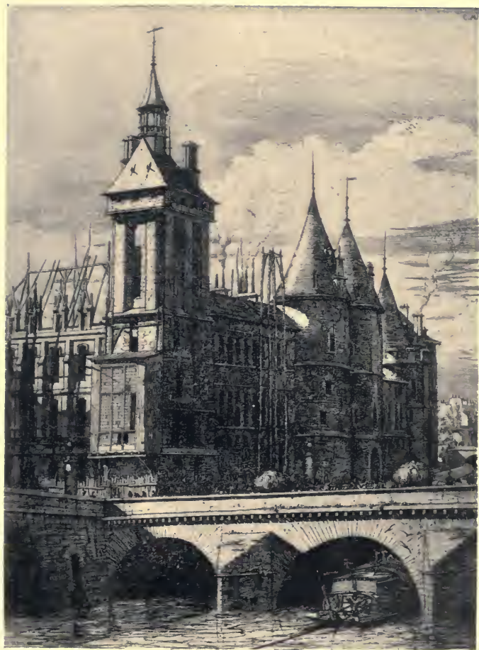
THE "PALAIS DE JUSTICE" AND TOWERS OF THE PRISON OF THE CONCIERGERIE
